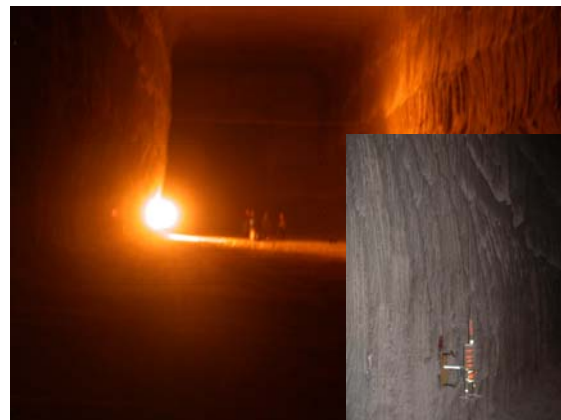
Fig.2. Photo of the existing big salt cavern; inset shows an element of the measuring system used for the long term monitoring of wall movements due to salt viscous creep.
